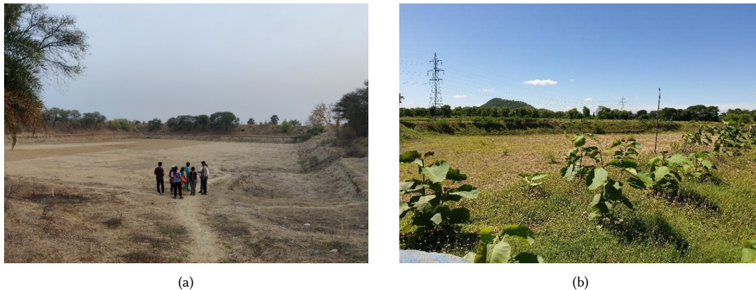
Fig. 1. (a) Farm pond built over a lineament. Lineaments are faults in the Earth's crust that can aid water infiltration to deeper aquifers, thus lowering the water retention capacity. (b) A poorly built farm pond, on a flat stretch of land with no inlets or outlets. Sections of boundaries were incomplete.
